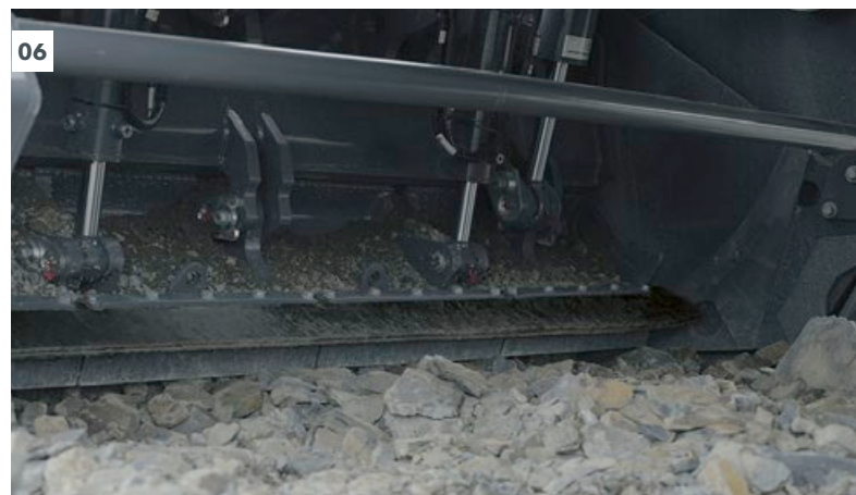
04 Coarse rocks build up in front of the active front door. 05 The active front door is opened manually and the material is pushed into the crushing and mixing housing as the machine advances. 06 The active front door is closed to minimize the ejection of material towards the front.
