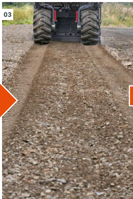
03 Crushing and mixing result: assess and if necessary adjust the parameters
