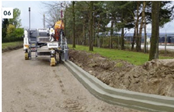
01 Special "parapet" application for safety barriers that are extremely difficult to penetrate: both right-sided paving ... 02 ... as well as left-sided paving of concrete safety barriers with continuous reinforcement. 03 Producing footpaths and bicycle paths up to 5 ft 11 in (1.8 m)* - seen here with a modularly extendable mold. 04 - 05 Production of small and large water gutters. 06 Precise production of curb / gutter profiles using AutoPilot 2.0. 07 Paving a slot drain for rainwater drainage.
