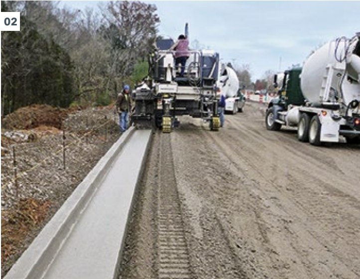
01 Software developed in-house guarantees maximum operational safety. 02 - 03 The high-quality machine control system ensures that the machine can travel both perfectly straight and precisely around curves. 04 Separate valves on all crawler units for high-precision control of height adjustment and steering.
