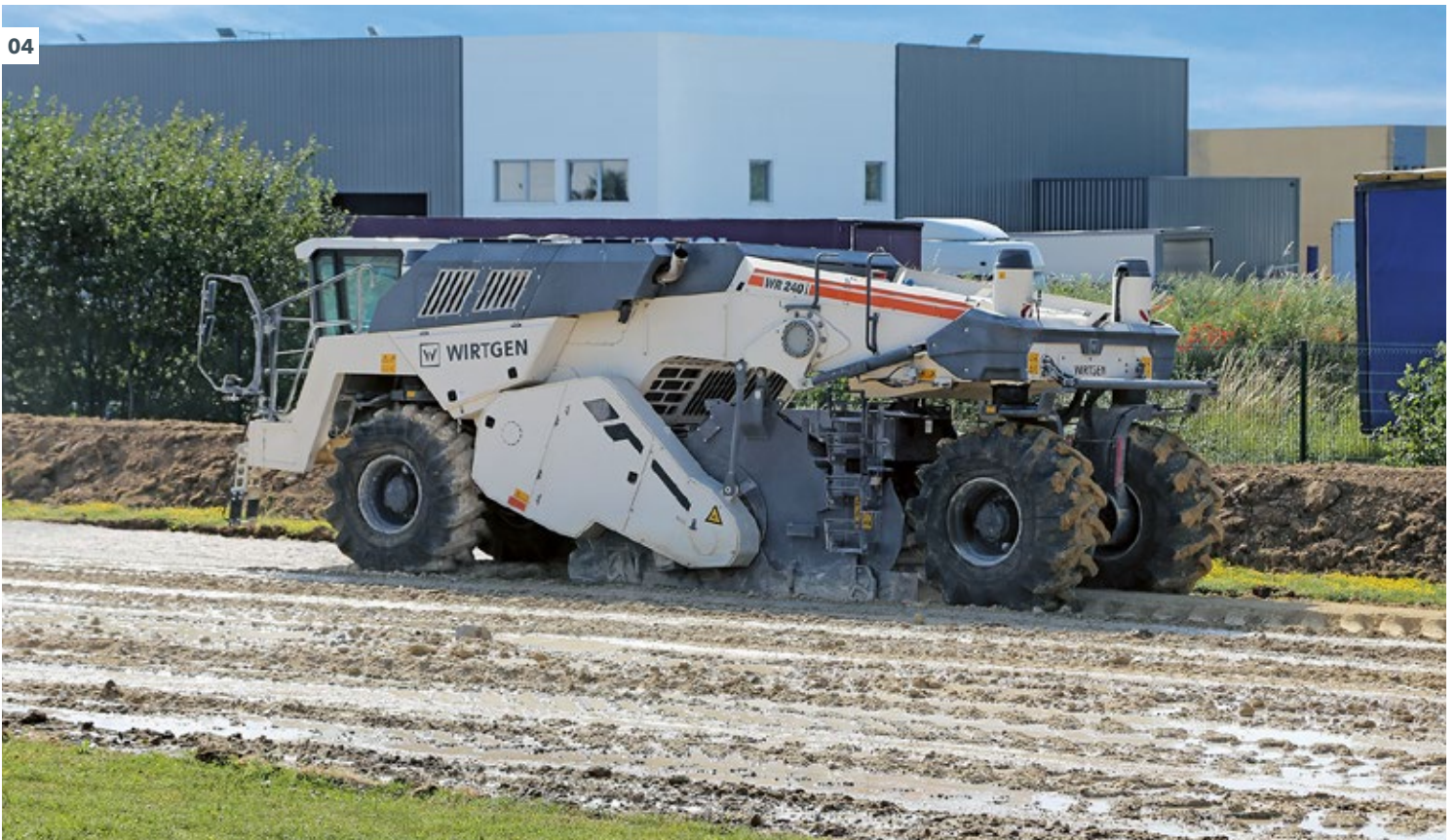
01 - 04 Soil stabilization involves transforming sub-bases with insufficient bearing capacity into soil that is perfect for paving and compaction.
