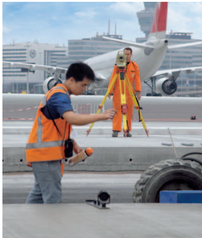
Verification measurements during the paving operation showed that the SP 1600 worked with maximum precision: Level and slope of the concrete surface precisely matched the specified requirements.
