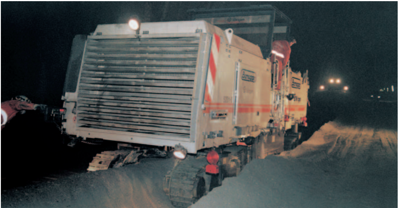
The cut, small-sized material was placed in a windrow behind the Surface Miner. Wheel loaders can easily pick it up and load it onto trucks.
