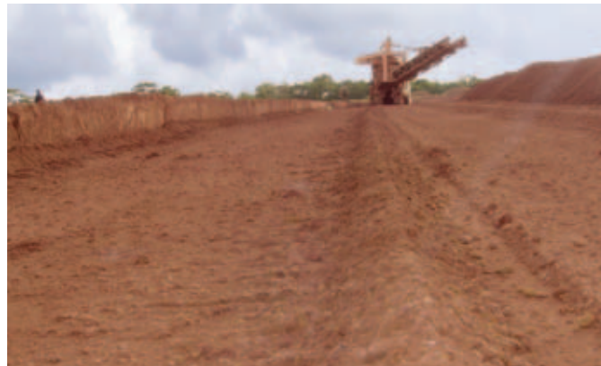
Surface Miners are able to mine materials with varying hardness without interrupting the mining process.
