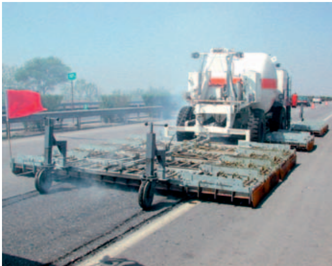
The Wirtgen HM 4500 Preheater heats the asphalt ahead of the remixer.
