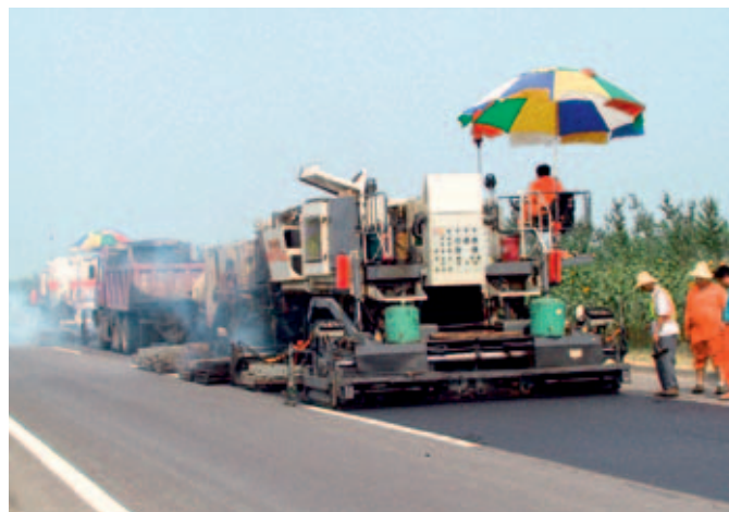
Remixing being carried out on the slow lane.
