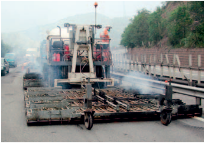
Hot in place recycling on the Cheng-Yu expressway, showing the preheater heating the old pavement as well as the newly paved asphalt behind the remixer.
