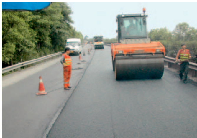
Second hot in place recycling project, on the Cheng-Yu expressway showing the compaction of the recycled asphalt layer using a Hamm HD 130 vibrating roller, as well as a view of the completed pavement.
