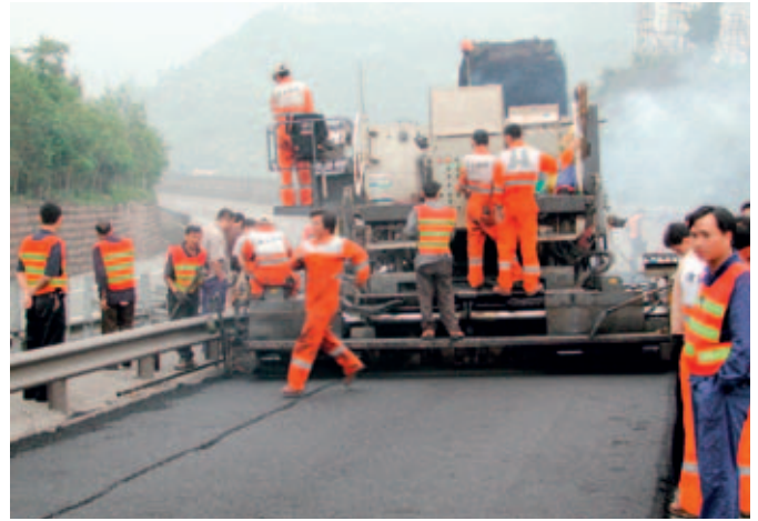
Hot in place recycling on the Cheng-Yu expressway, showing the preheater heating the old pavement as well as the newly paved asphalt behind the remixer.
