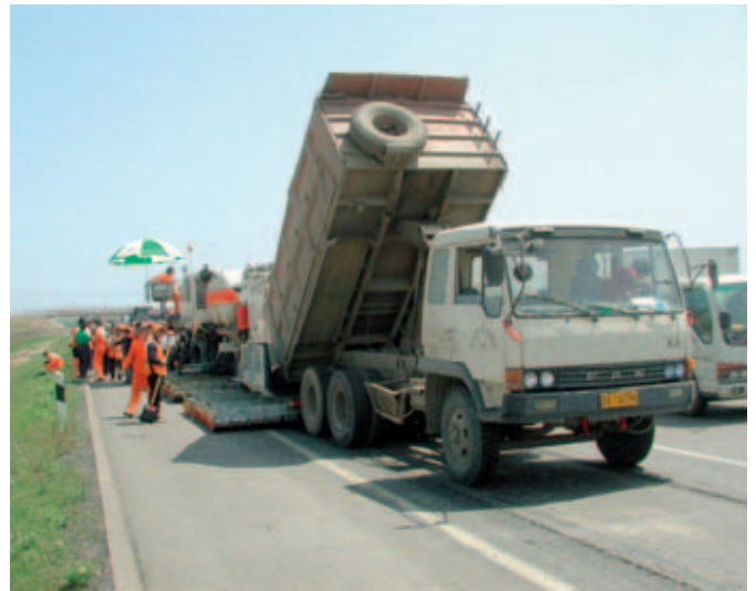
New asphalt mix being tipped into the Wirtgen Remixer RX 4500.
