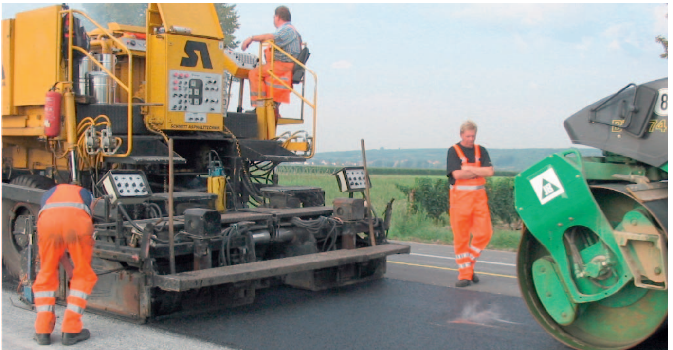
Fig. 12: Placement and final compaction of the mix.
