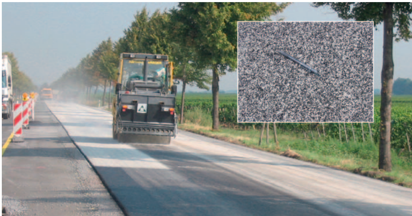
Fig. 14: Gritting of the asphalt surface.
