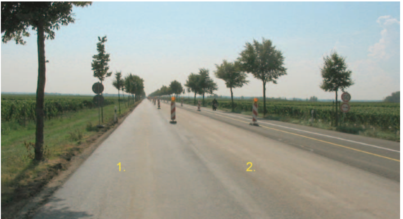
Fig. 16: Completed sections 1 and 2.
