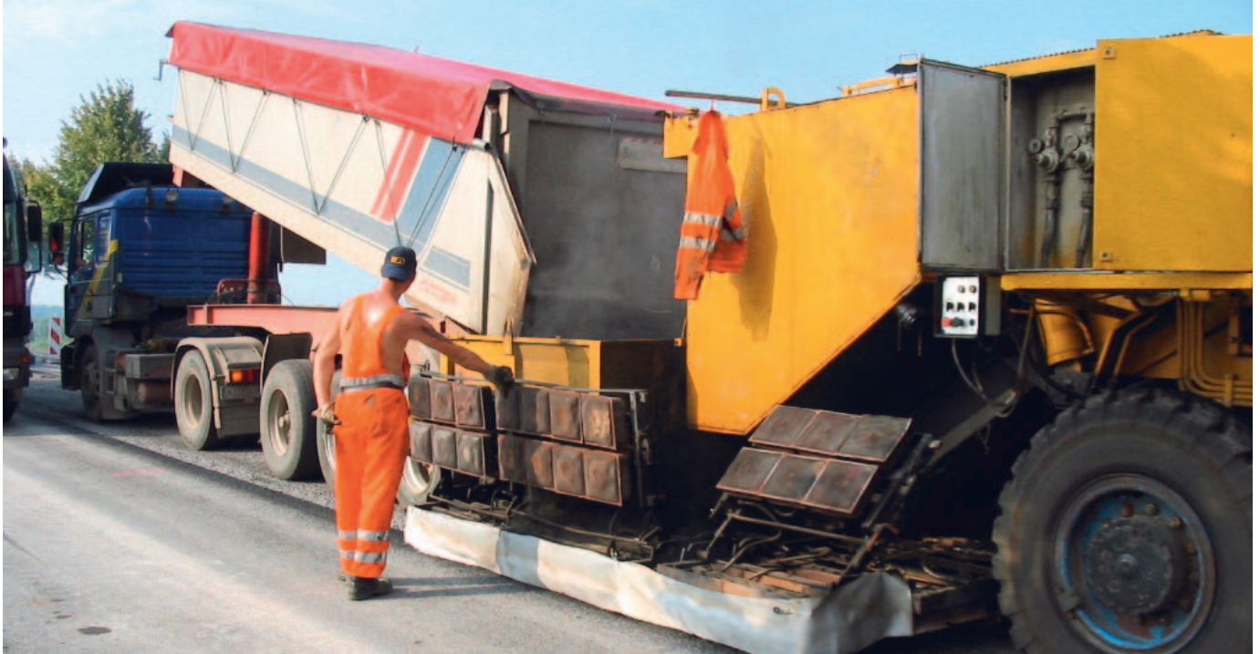
Fig. 8: Feeding of the Wirtgen Remixer 4500 with asphalt mix.
