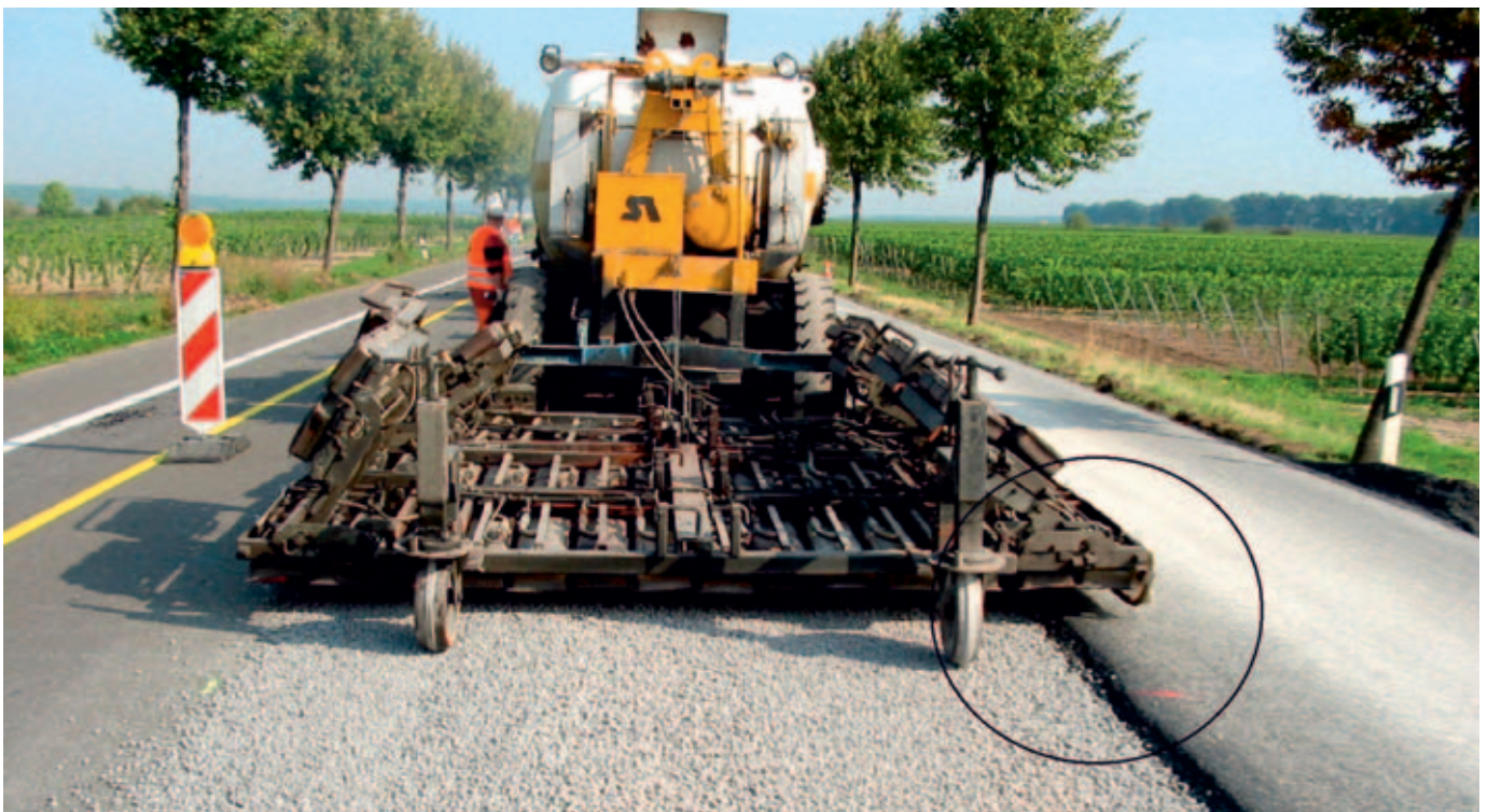
Fig. 5: The overlapping heating of the roadway ensures a seamless joint.
