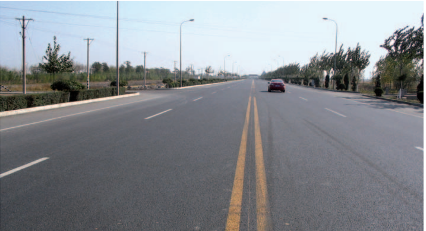
The final surface after the last surfacing process.
