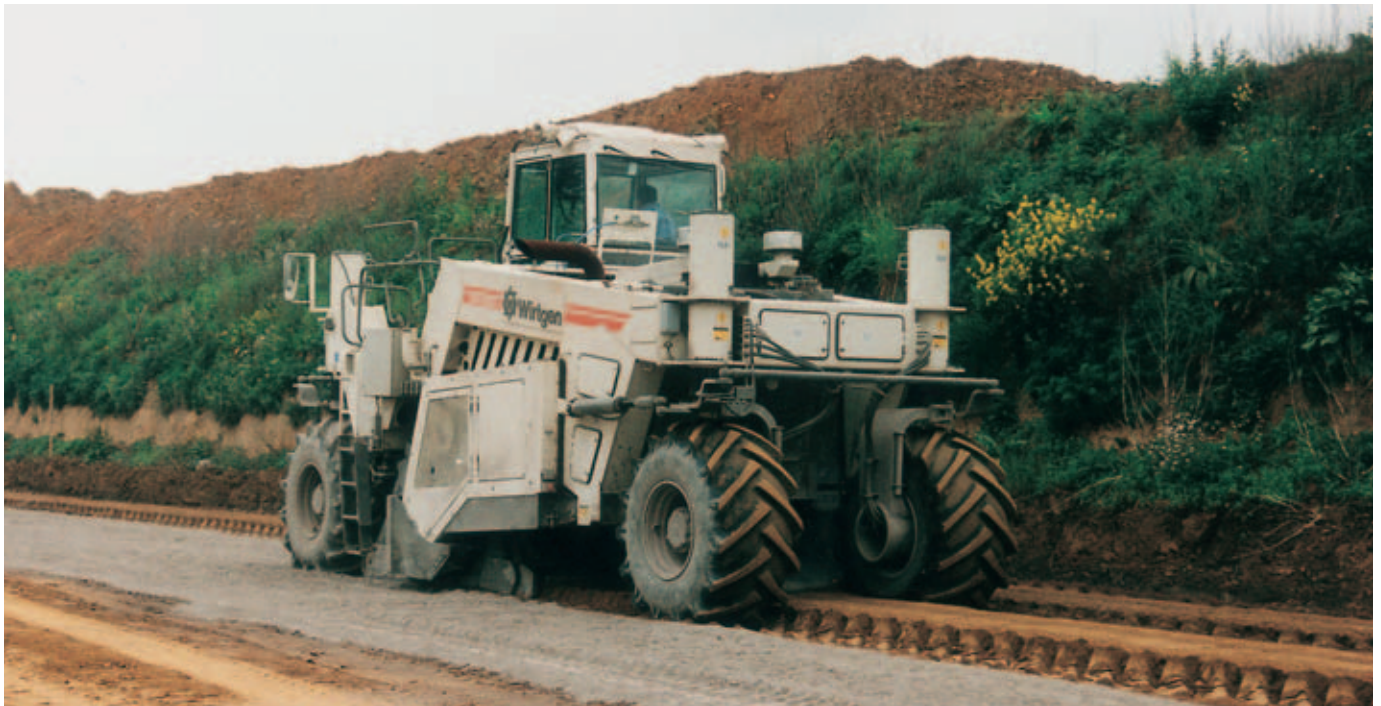
High performance when soil solidificating with cement near Wiesbaden.
