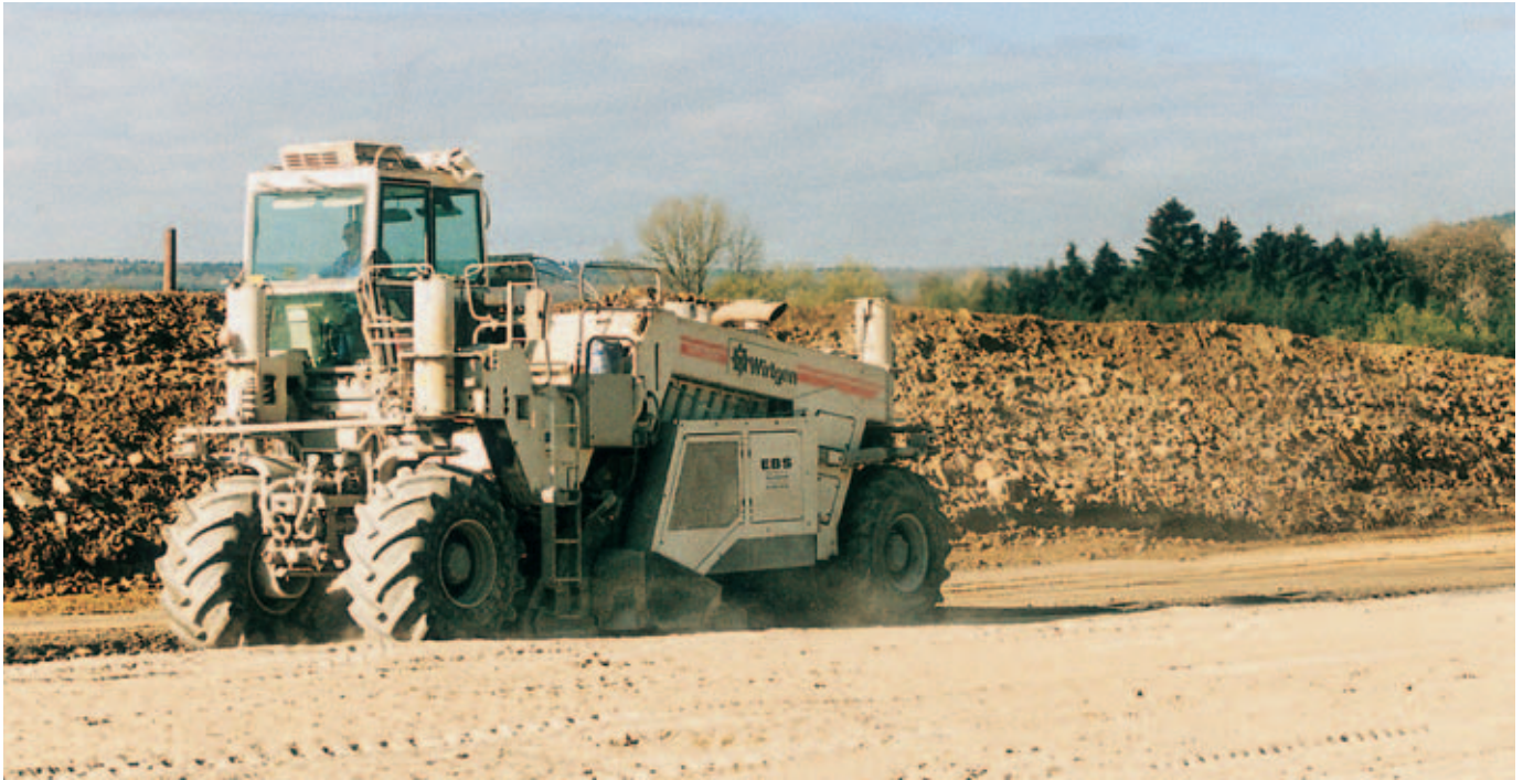
Soil stabilizing with Terrafox for building the new railway station Montabaur.
