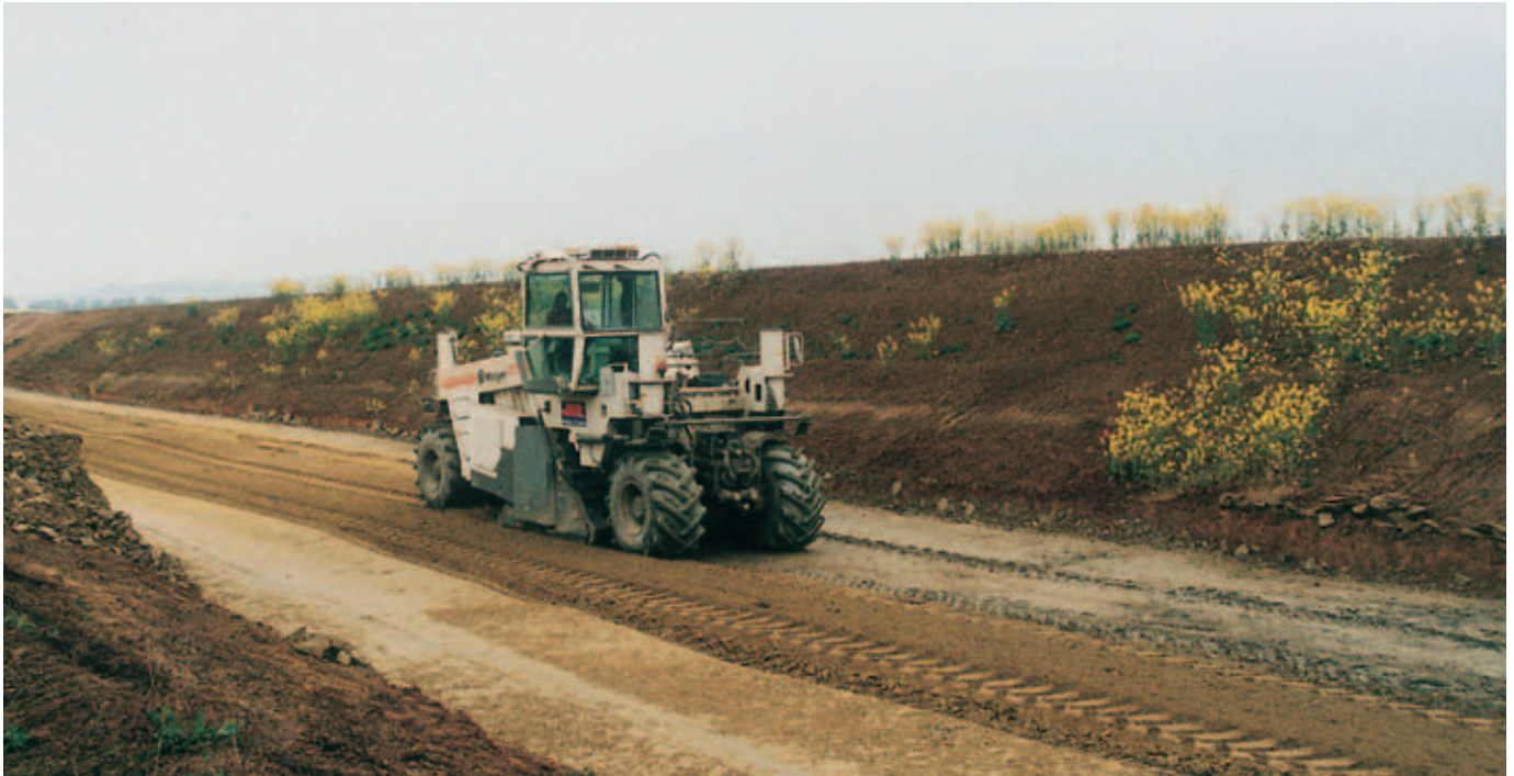
In two to three passes, this coarse aggregate is crushed to a maximum sieve size of 10 cm.
