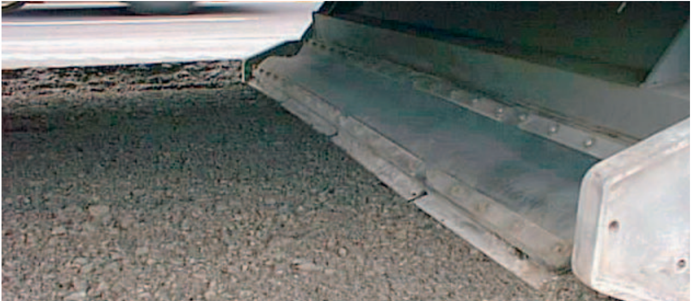
Fig. 7: The stabilised material viewed directly behind the milling and mixing chamber.
