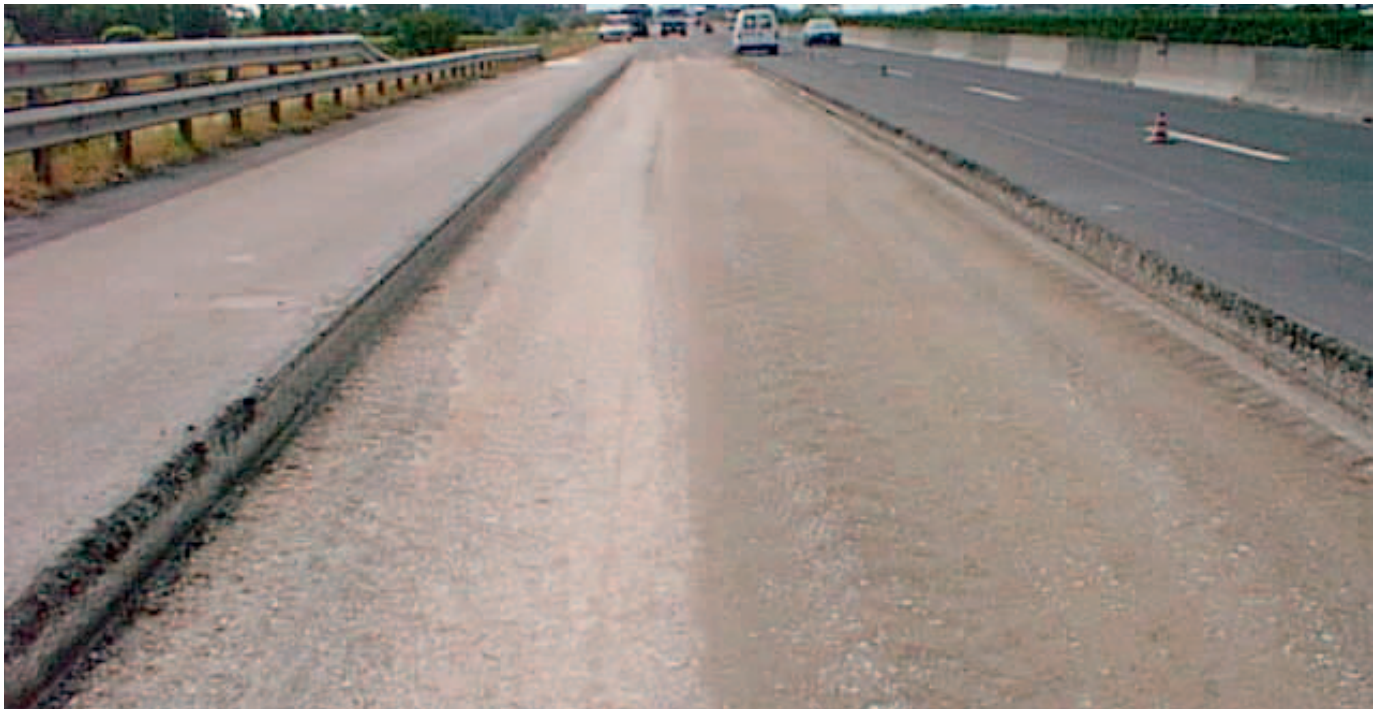
Fig. 11: The compacted and finished recycled layer.
