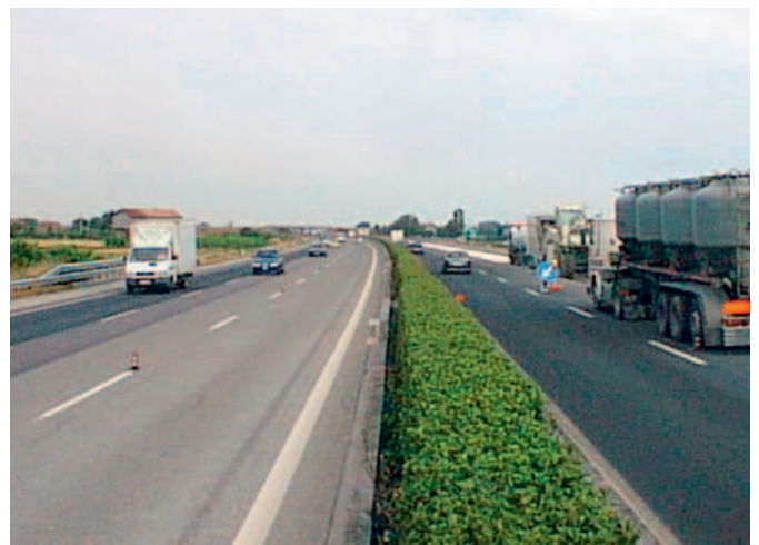
Fig. 13: This is being done on both the north and south-bound carriageway of the A14 between Bologna and Rimini.
