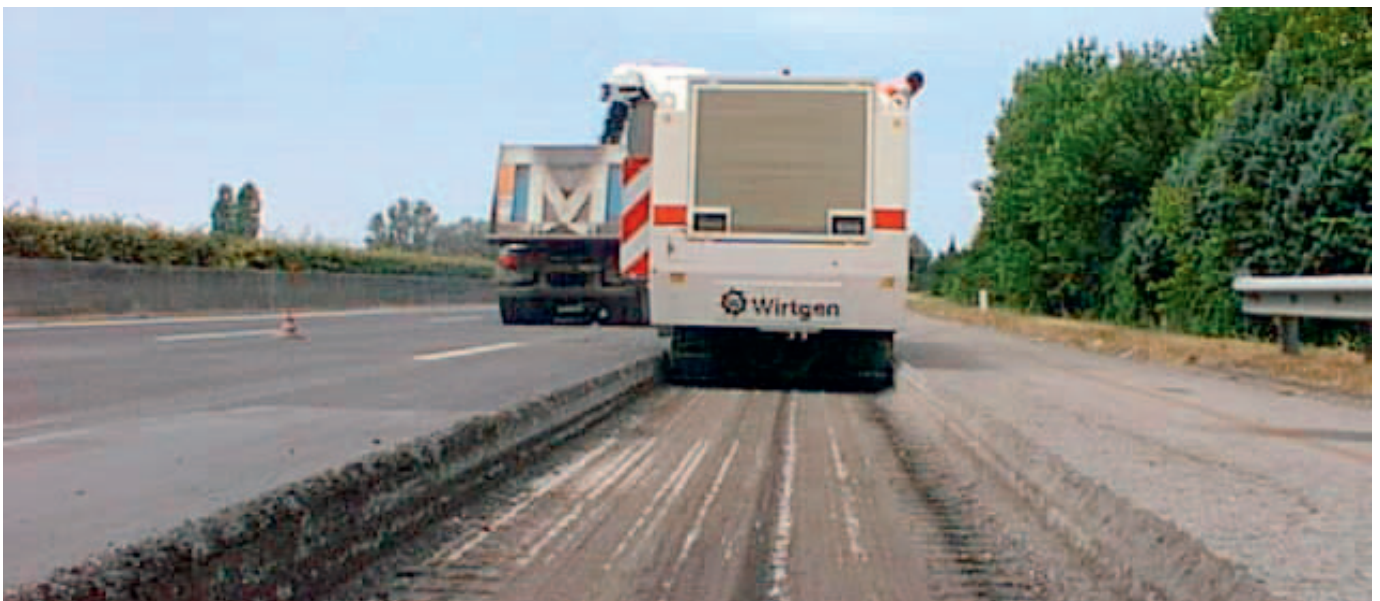
Fig. 4: The first 28 cm deep and 2,1 m wide milling cut using a Wirtgen 2100 DC.
