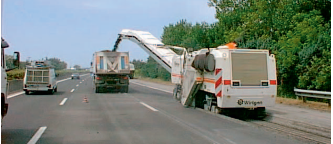
Fig. 3: The Wirtgen 2100 DC loading the milled asphalt directly onto a truck.
