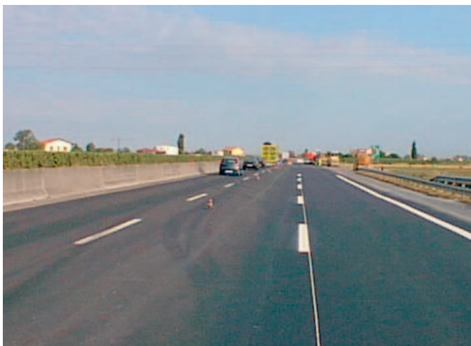
Fig. 12: A view of the finished asphalted and line marked slow lane, ready for the heavy traffic.
