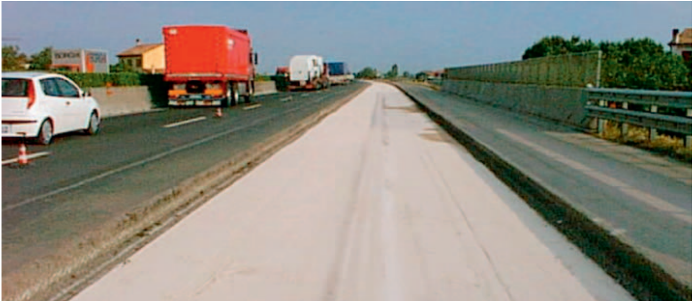
Fig. 5: 0/2 mm crusher dust spread to the 4 m wide milled out section.
