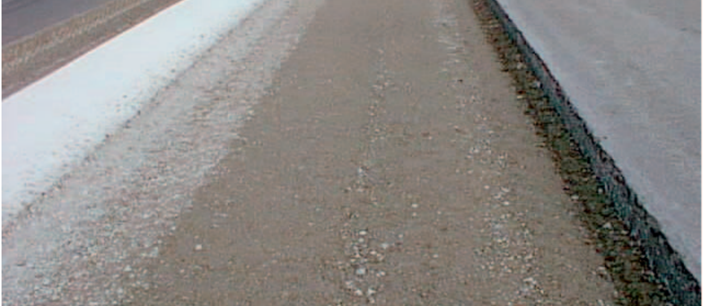
Fig. 9: The first pass compacted and finished.
