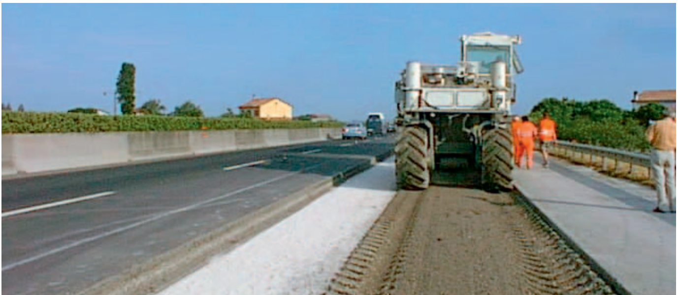
Fig. 6: First pass of the Wirtgen recycling train.
