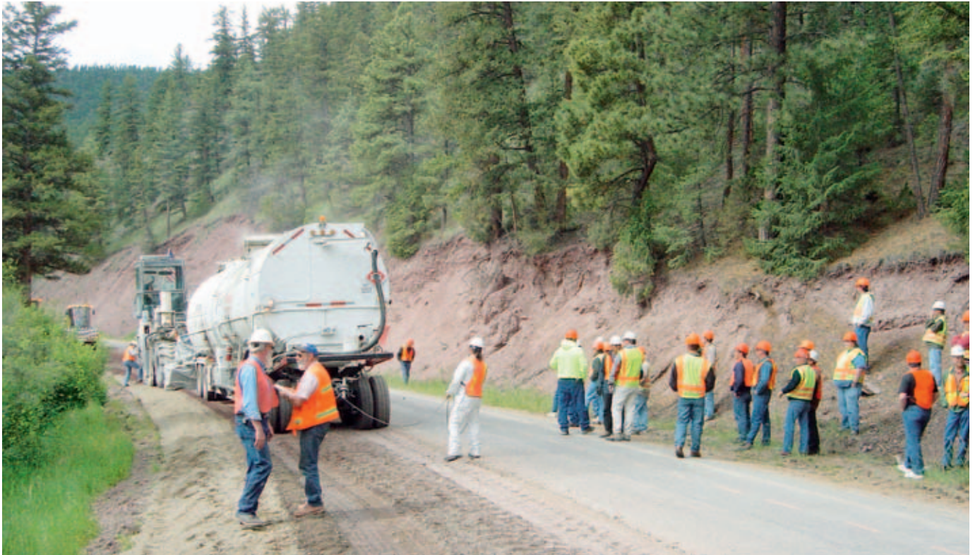
Visiting Engineers inspect the foamed asphalt base stabilisation process.
