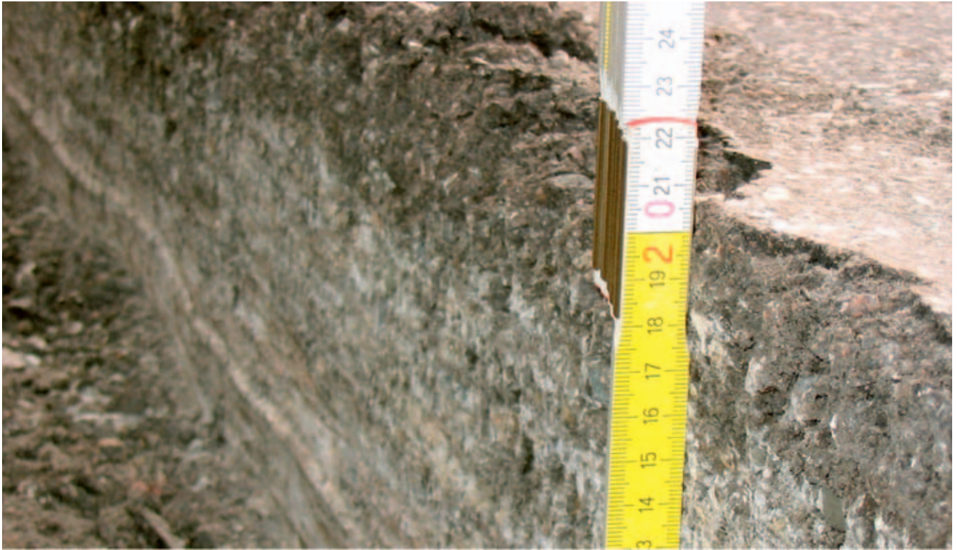
20 cm of asphalt in the existing pavement.
