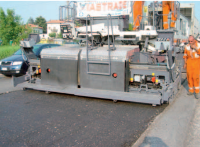
Vögele AB 500 tamping & vibrating screed, set to 3,800 mm paving width.
