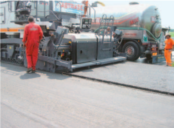
Recycling / paving speed: Average 3,20 m per minute.
