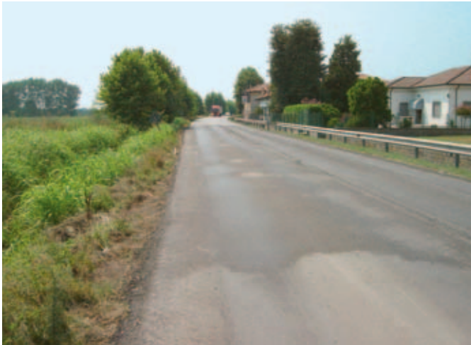
Finished compacted recycled lane prior to traffic.
