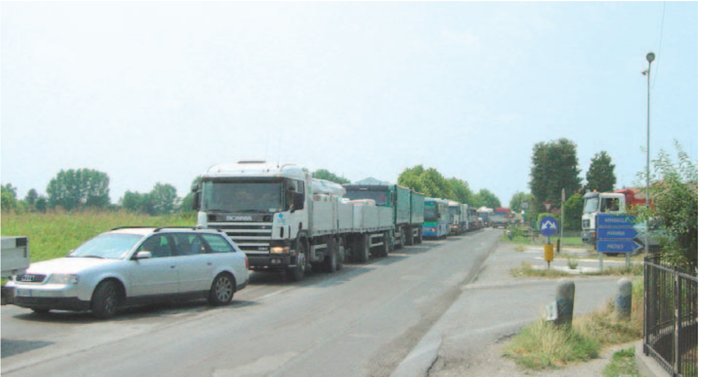
Traffic using recycled lane within 3 hours of recycling.
