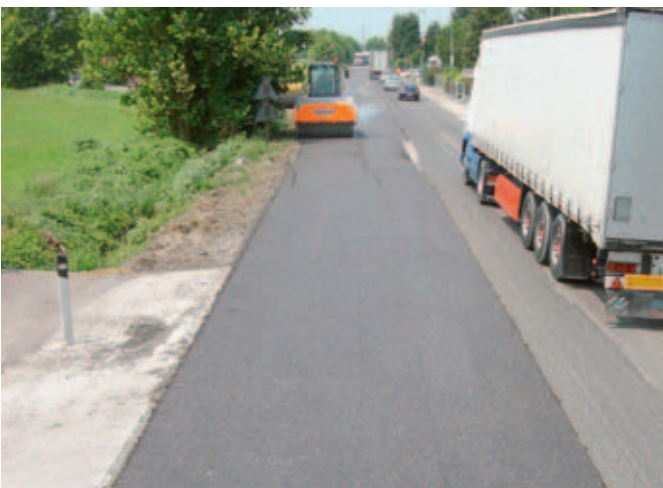
Average paving 345 tons per hour.
