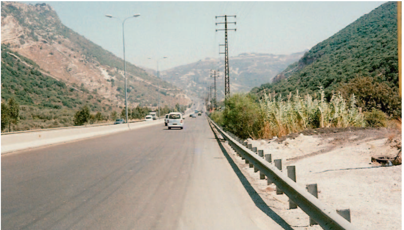
The rehabilitated highway with the asphalt overlay.
