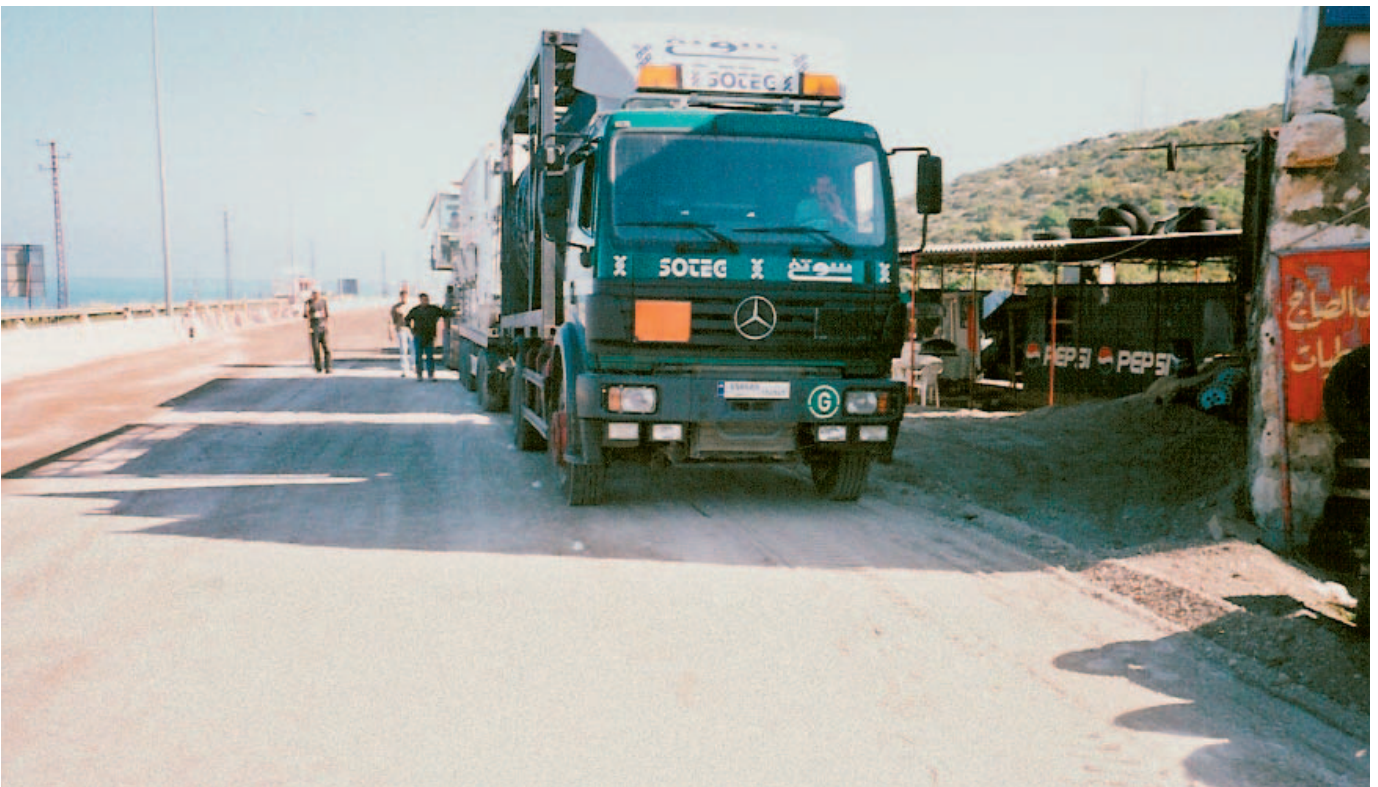
Spreading fines to modify the gradation.
