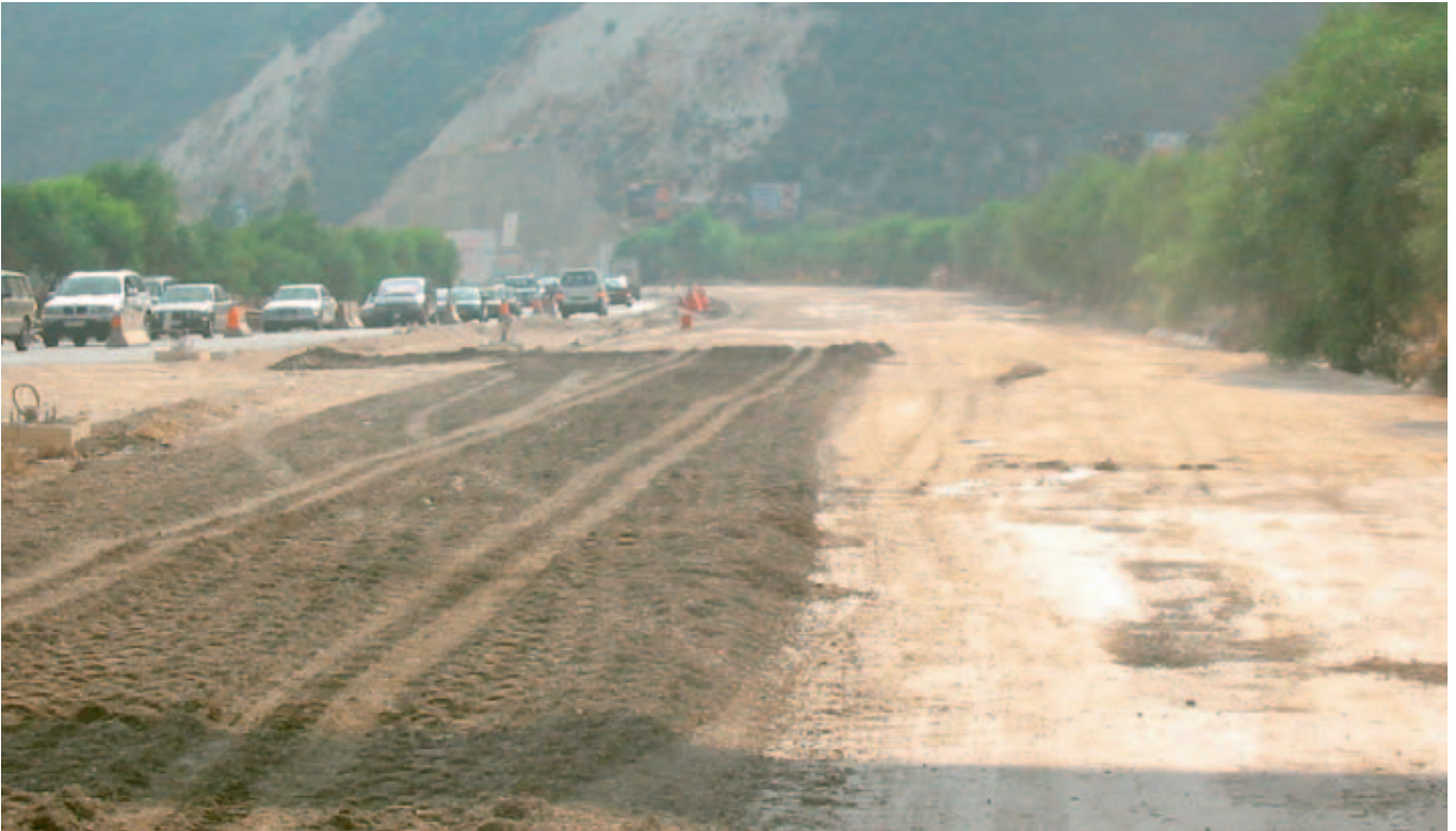
Spreading the recycled material to get the required profile.
