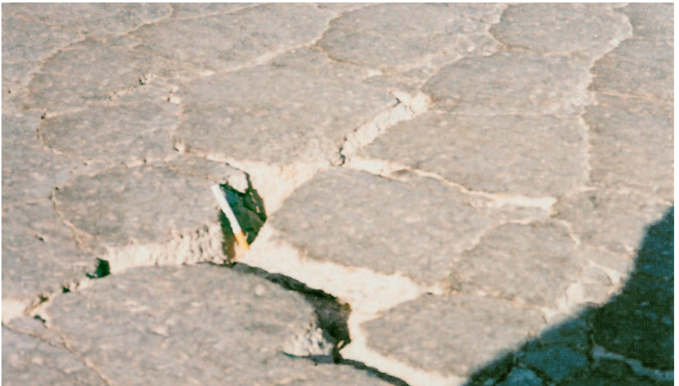
Typical pavement condition prior to recycling.
