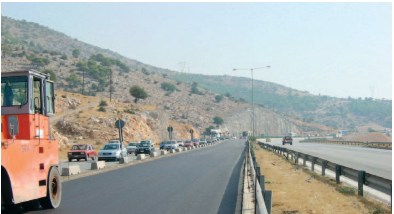
The outer half of the carriageway is then recycled.
