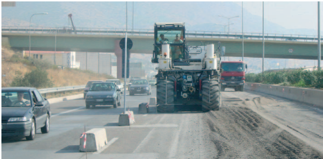
Prepulverising with the Wirtgen WR 2500 S.
