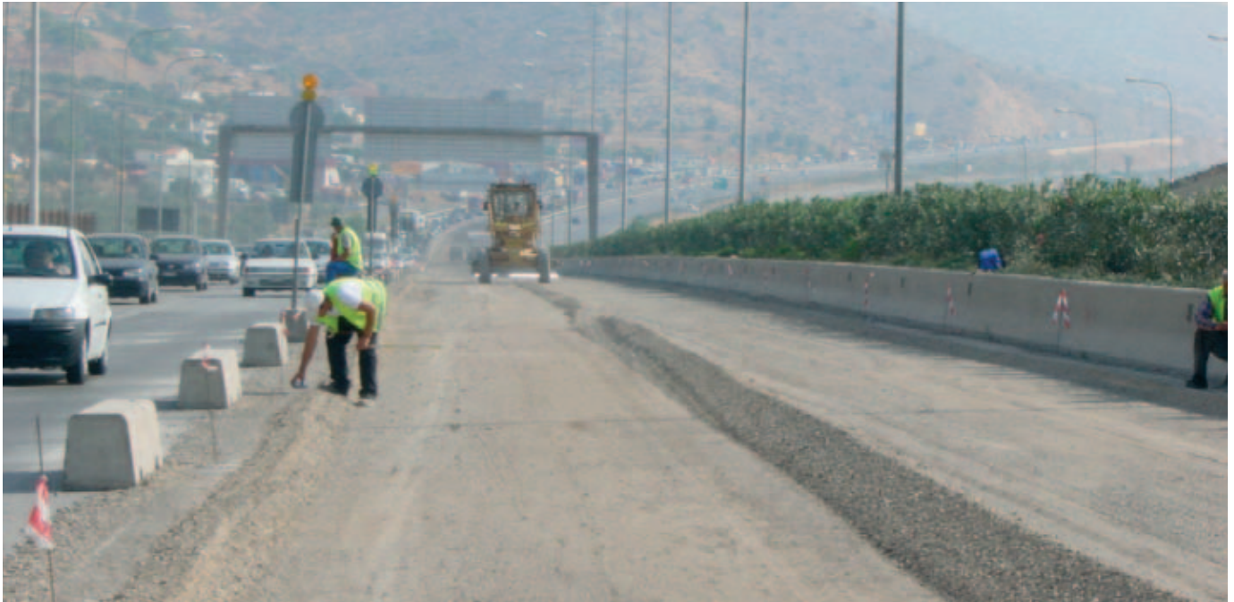
Cutting surface levels prior to stabilising.
