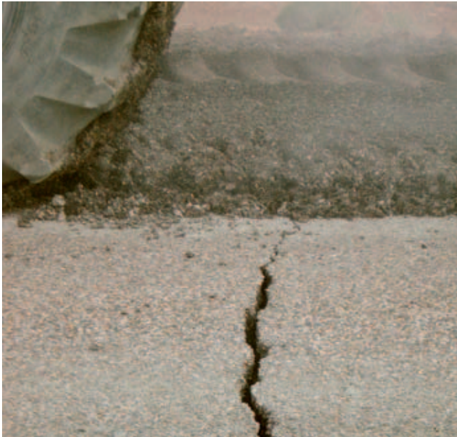
The recycler cuts through the asphalt into the base eliminating the crack.
