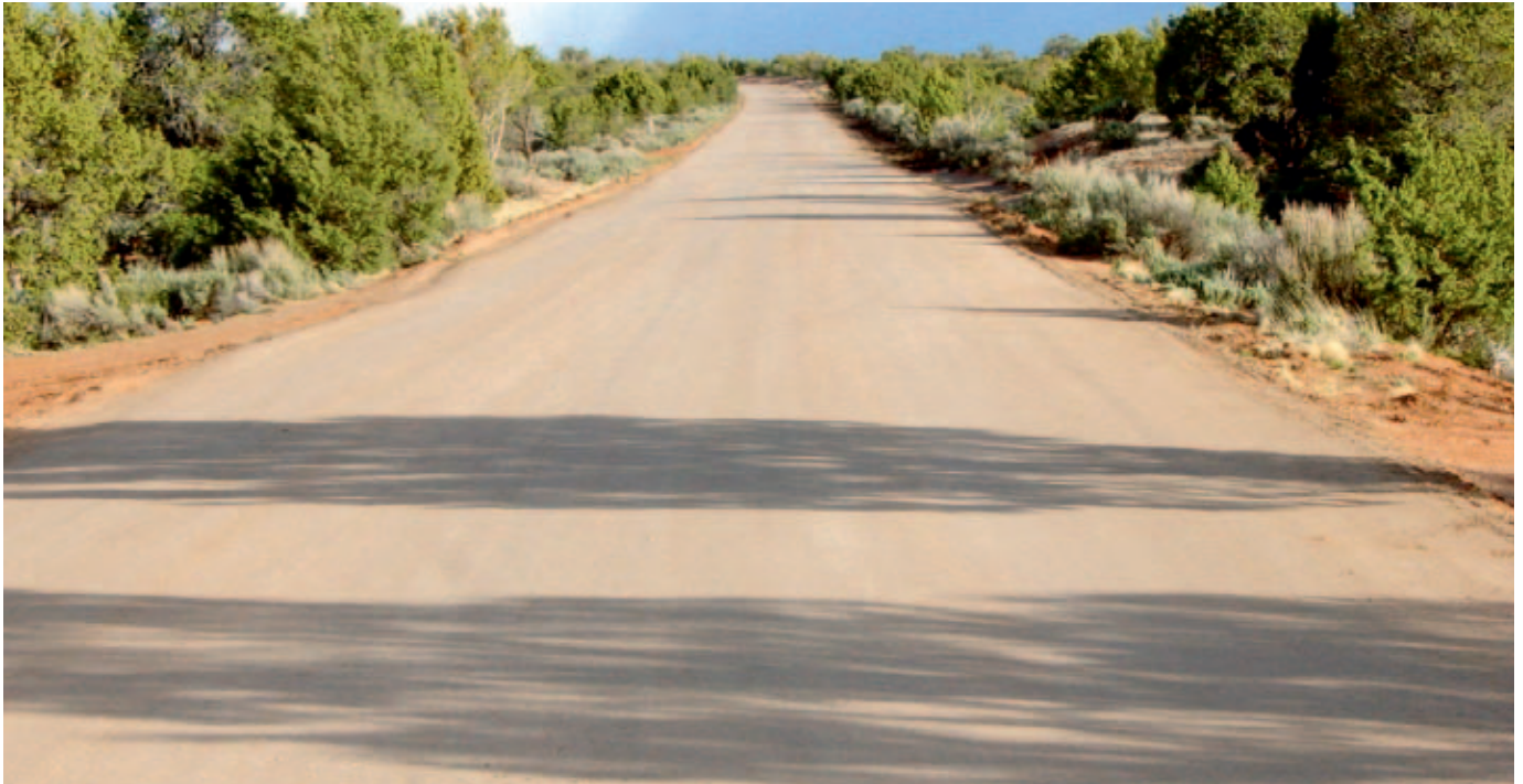
Recycled pavement finish shaped and compacted prior to overlay.
