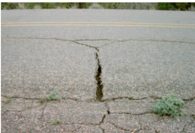
Typical views of the pavement condition prior to recycling.
