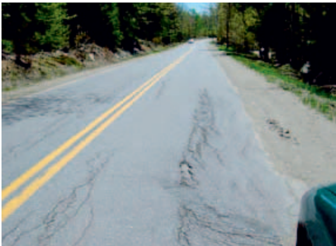
May 2001 Route 8 mid section looking south
