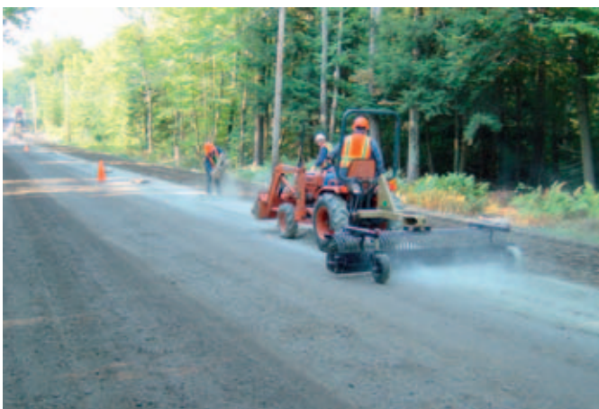
The cement was initially laid out by hand.
