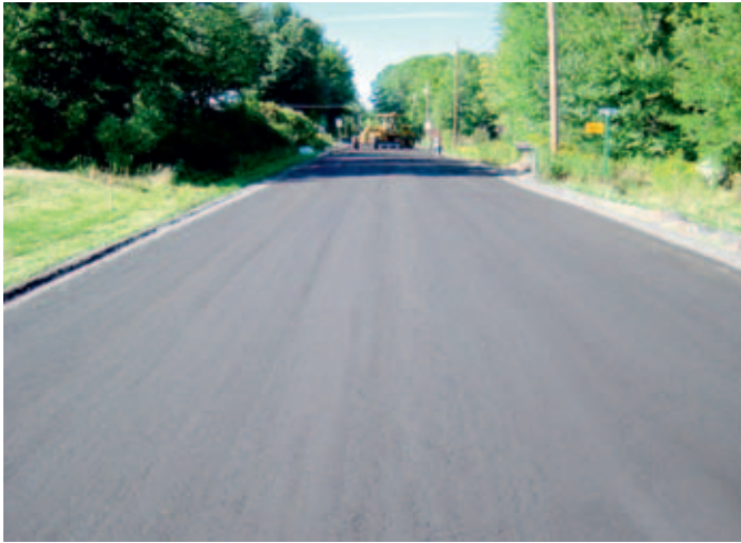
Finished foam stabilized base
