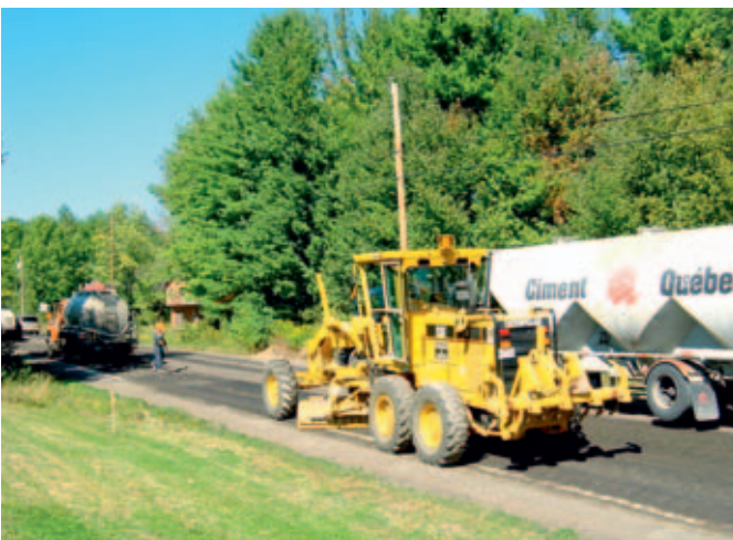
Cut levels with motor grader
